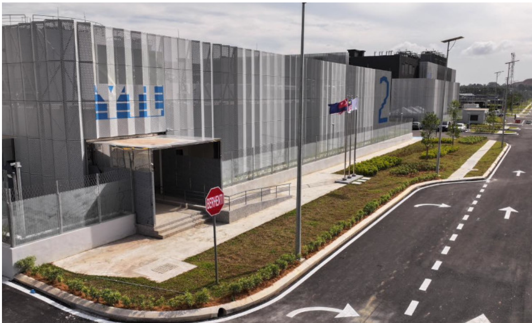
Photo: Property exterior: YTL Johor Data Center Park. [4]
