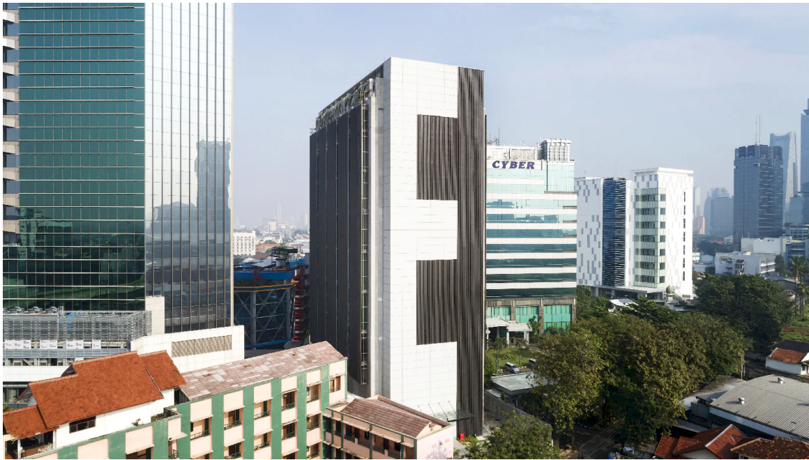
Photo: Property exterior: Digital Edge EDGE1. [3]
