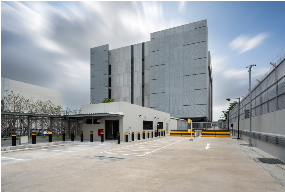
Photo: Property exterior: GSA01. [3]
