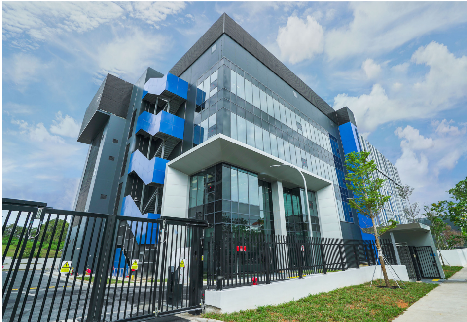
Photo: Property exterior: Digital Realty SIN12. [3]
